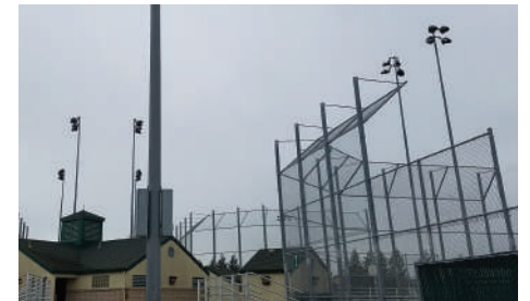
View of the baseball/softball field backstops and stadium lighting.
